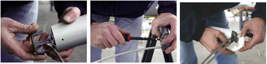
Check the positioning of the cables before fixing the tips of the spreaders
